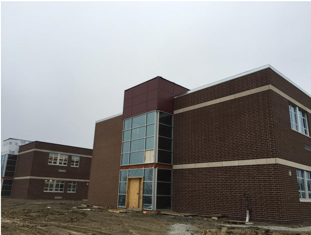
Area B siding
