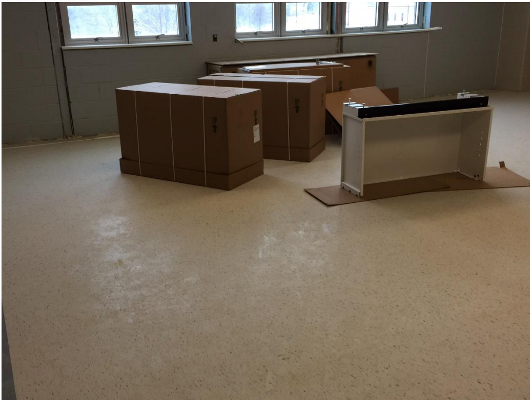
Metal casework for classrooms
