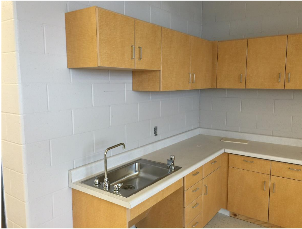
Kindergarten Classroom sink
