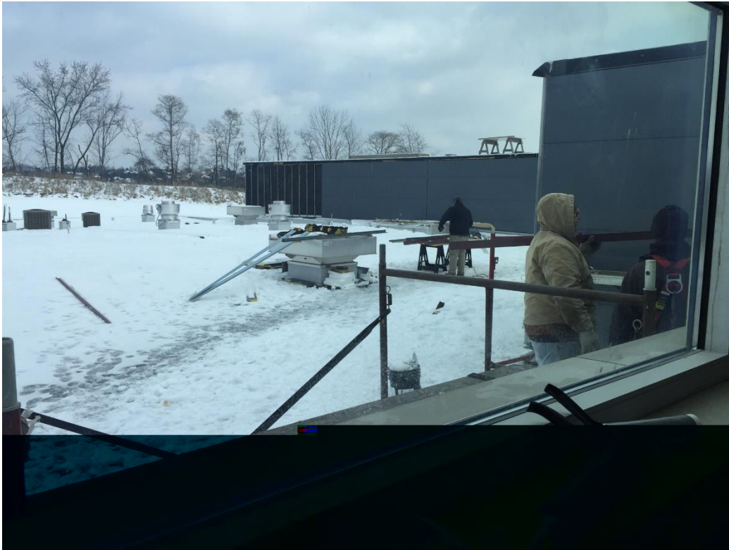
Area C siding
