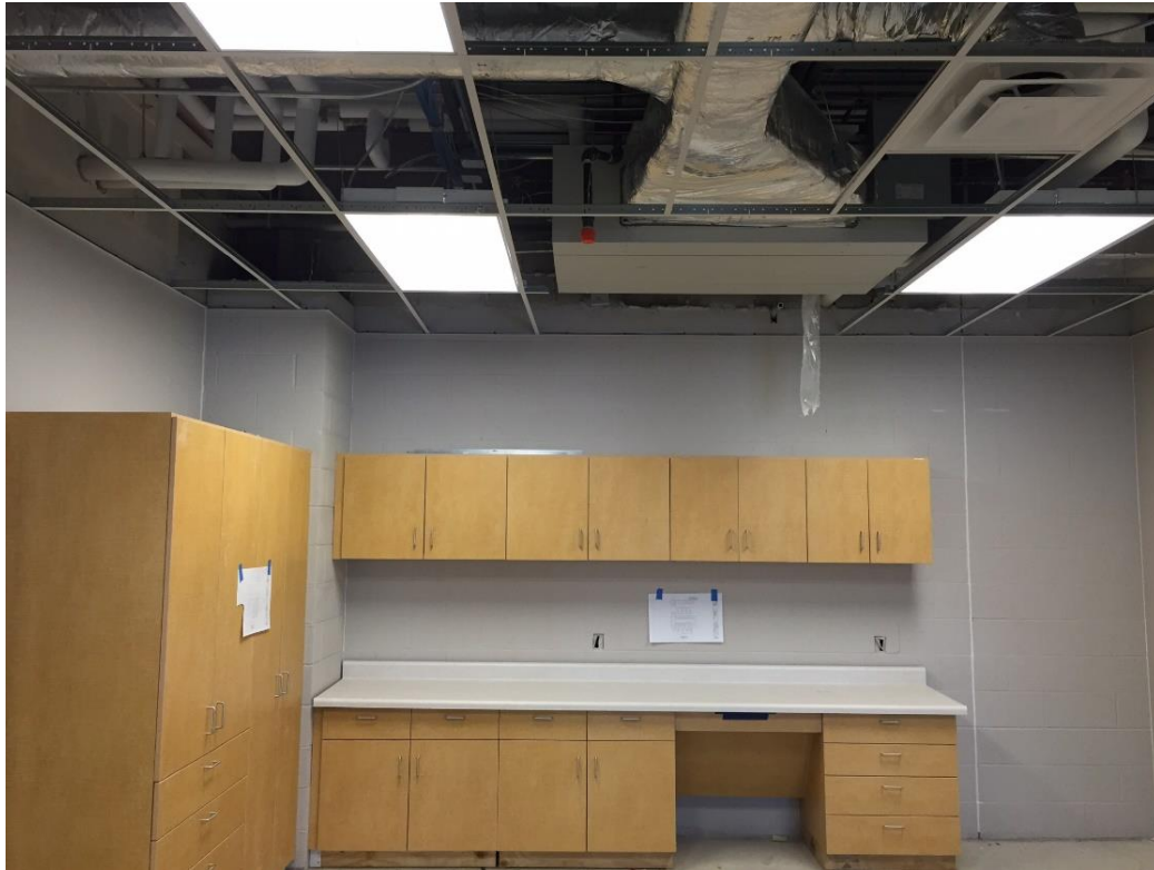
Principal office lighting and casework
